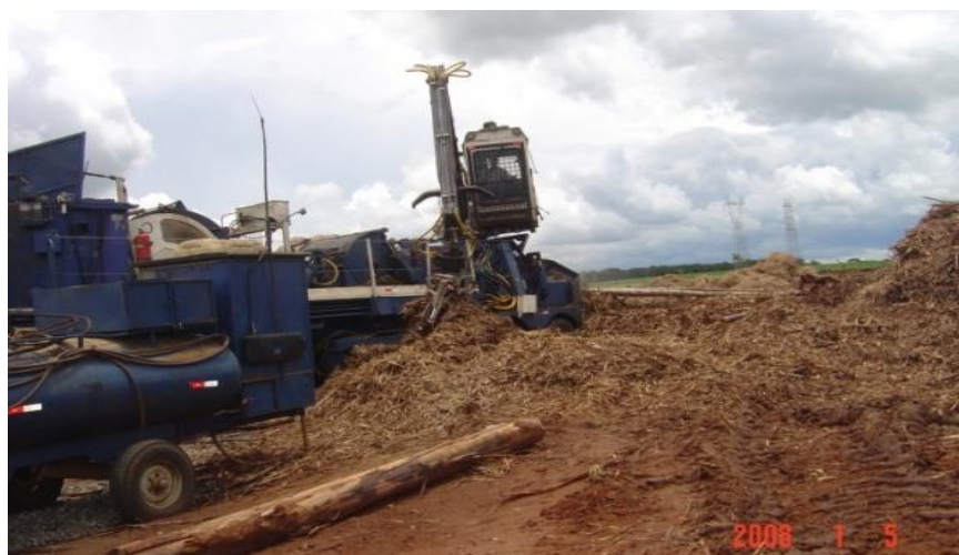
Figura 11 Limpeza material residual
